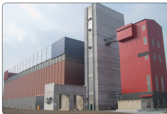
Silo de report
